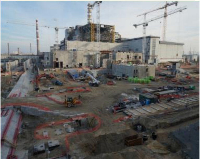
Transfer Zone Foundations North Strip
